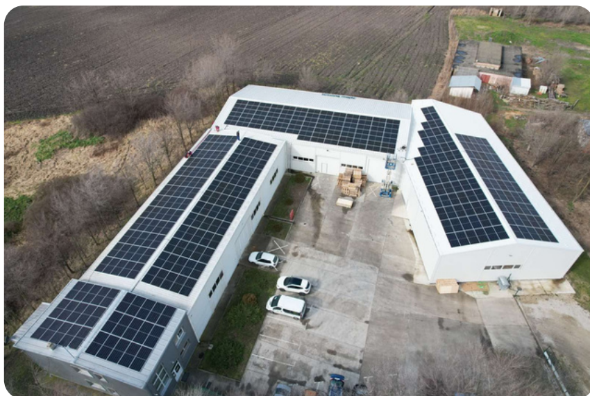
Polimer Commerce Plandište 200 kWp
